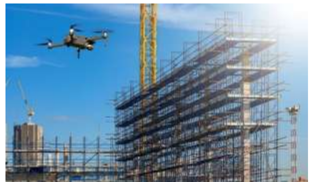
Fig .7 . Construction with UAVs and GNSS
