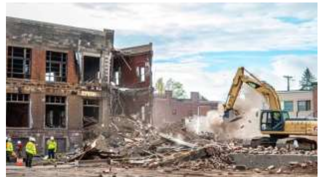
Fig: Traditional Demolition Scene
