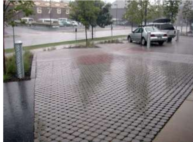
Figure 5: Permeable Pavements
