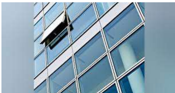
Figure 3: Operable Windows and Ventilation Openings
