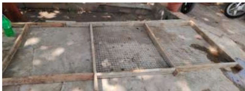
Fig.6.1 Ferrocement panel using steel
