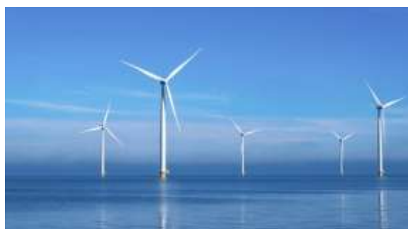
Fig .3 . Innovations in Offshore Renewable Energy
